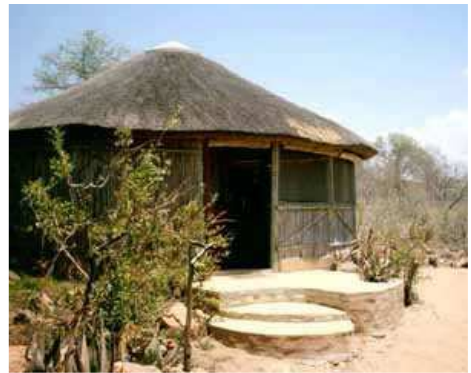
Sleeping hut, done in a simple gum pole and thatch construction but with great taste and attention to detail
