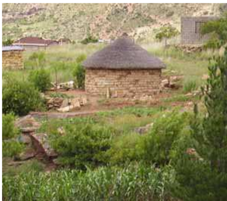
Round hut in nicely dressed stone masonry
