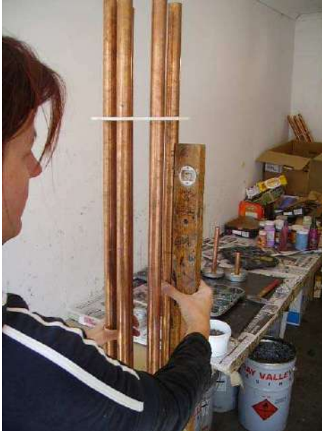
Make sure the pipes are level
