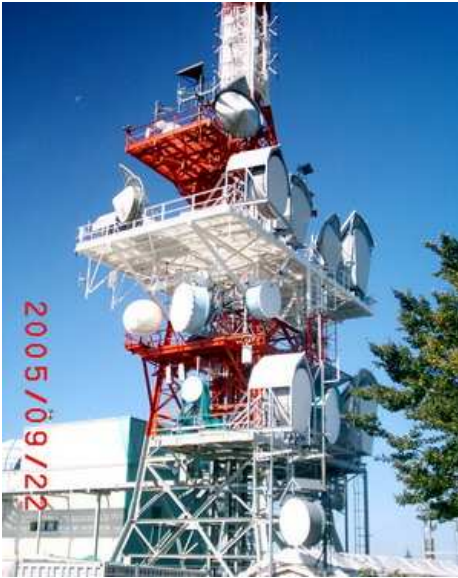
Massive entropy transmitter station on the Geißberg
