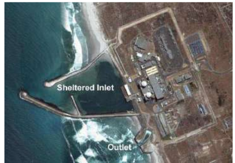
Aerial photo of Koeberg power station
