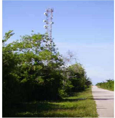
Transmitter site on the north-eastern coast
