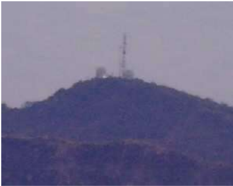
Hilltop array above Tete (Mozambique)
