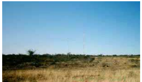
Transmitters along Transkalahari Highway
