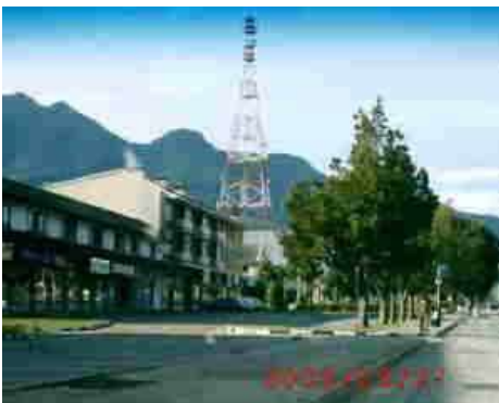
This tower was the culprit
