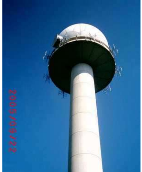
This also stands near the Kaiserbuche, now surrounded by TBs
